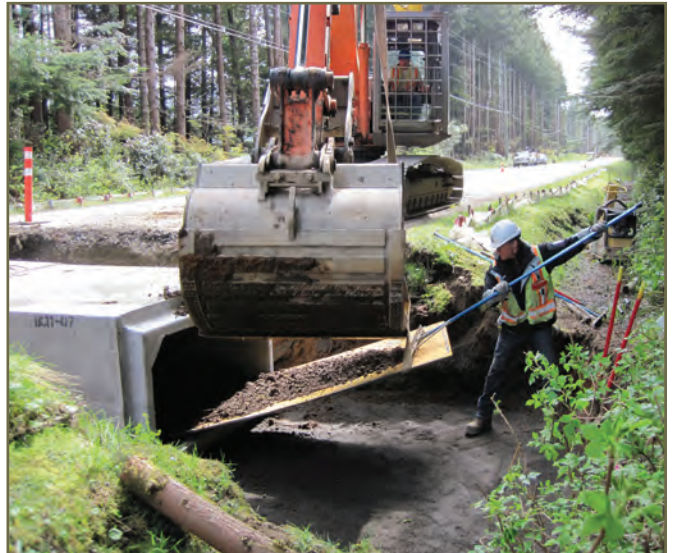
Photo 12. Adding soil to box tunnel near Ucluelet, B.C. © Barb Beasley
