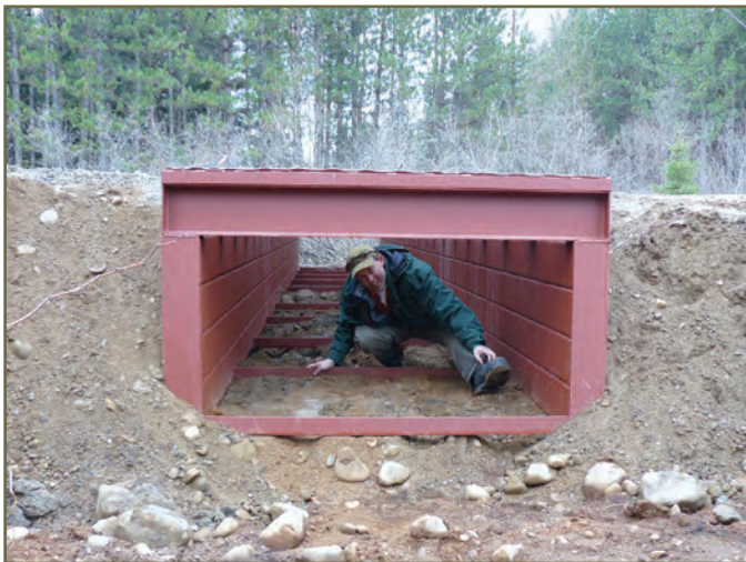
Photo 36. Tunnel structure with sediment baffles at bottom © B. Steinberg
