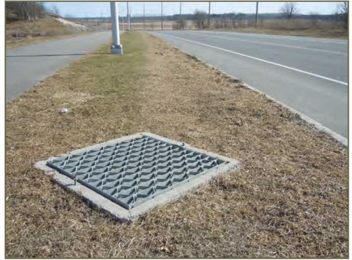
Photo 28. Open grate skylight in median on Terry Fox Extension, Ottawa, Ontario. © D. Seburn
