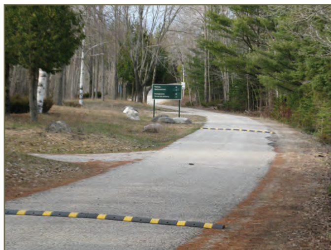
Photo 56. Speed bumps used to reduce speed on Cyprus Lake Road, Bruce Peninsula, Ontario. ©K. Gunson
