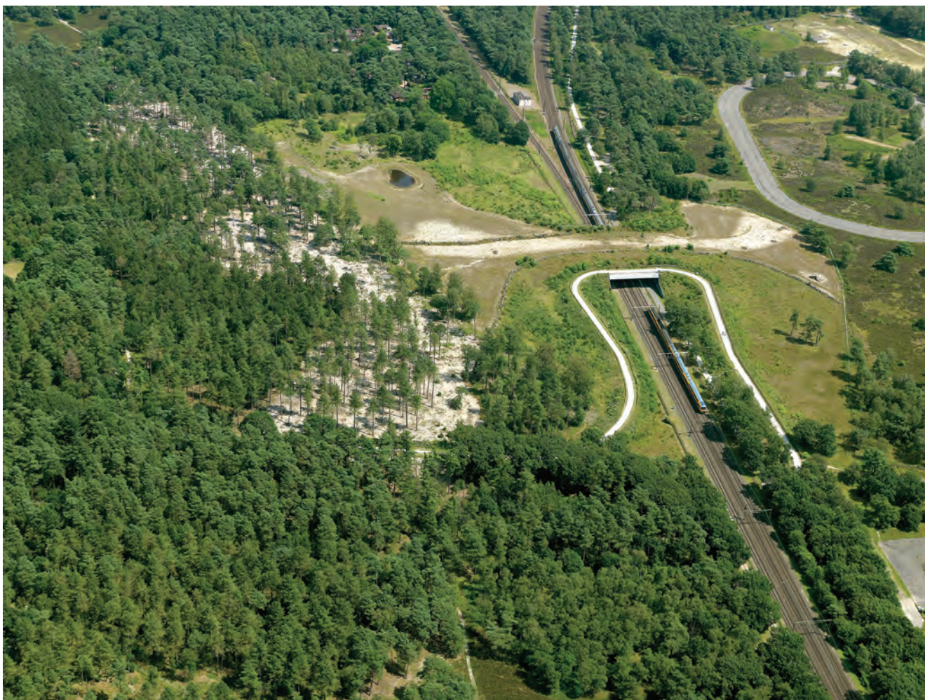
Figure 2. Ecoduct Op Hees, crossing the Utrecht–Amersfoort rail line. The recreation cycle path is situated at the foreground side of the bridge © ProRail
