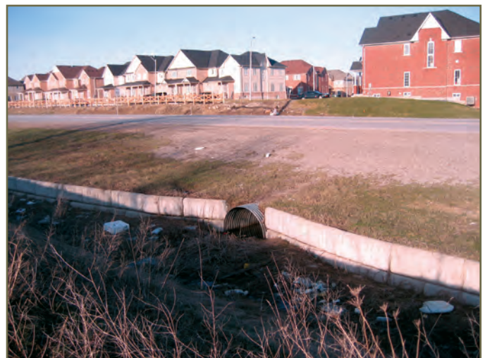
Photo 41. Concrete wall in Aurora, Ontario © K. Gunson
