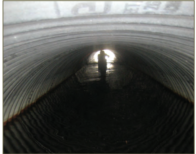
Photo 37. Large 1.8 m drainage culvert partially filled with standing water allows light into tunnel, Highway 24, Aurora, Ontario. © K. Gunson
