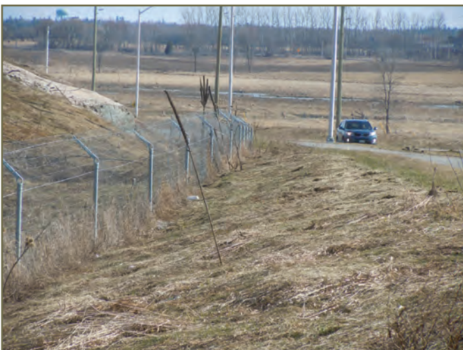
Photo 40. Chain link guide fencing and lip extension, Terry Fox Extension, Ottawa, Ontario © D. Seburn.
