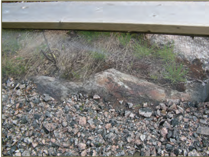
Photo 48. Fence along rock with gravel used to hold bottom of fence in place © K. Gunson
