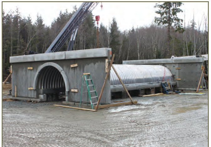
Photo 19. Arch culvert preassembled off site © K. Williams
