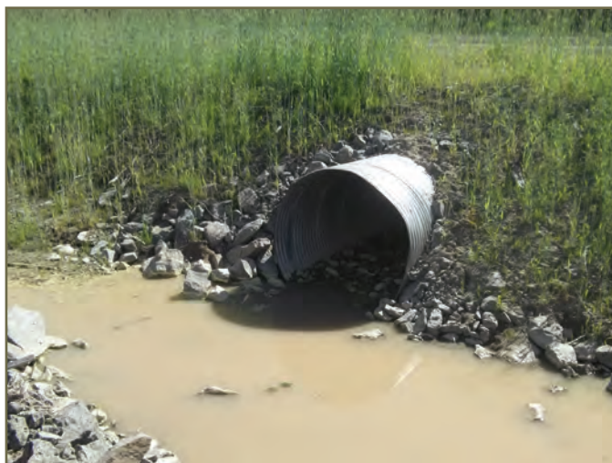
Photo 46. Pooling at culvert entrance that should be avoided at terrestrial wildlife tunnels © K. Gunson
