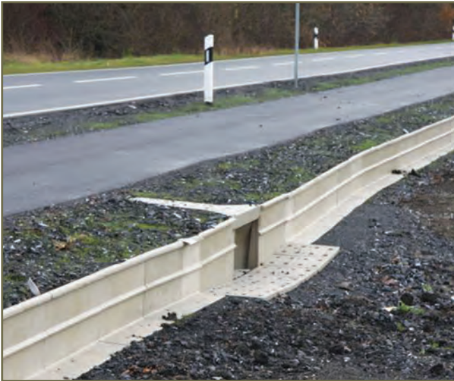
Photo 7. Open- and closed-top variation, Germany. © ACO International
